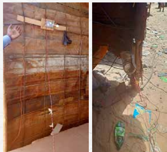
Hazardous electrical wiring
